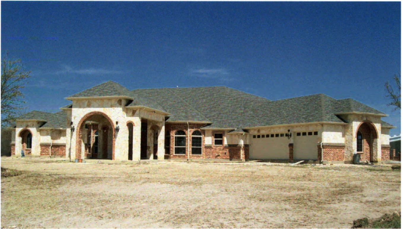
CLASS 5M VERY GOOD QUALITY MASONRY
