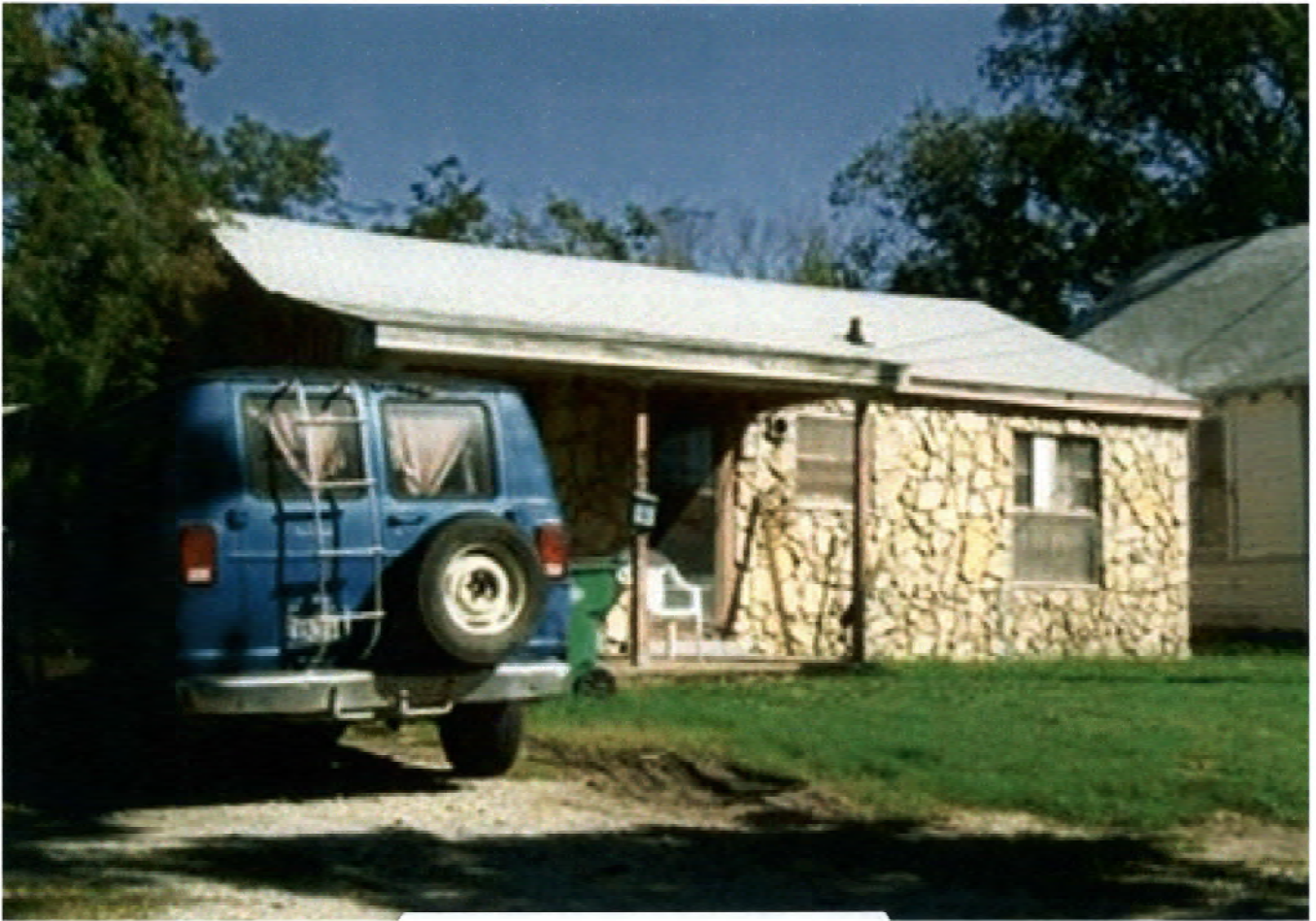
CLASS 1M LOW QUALITY MASONRY
