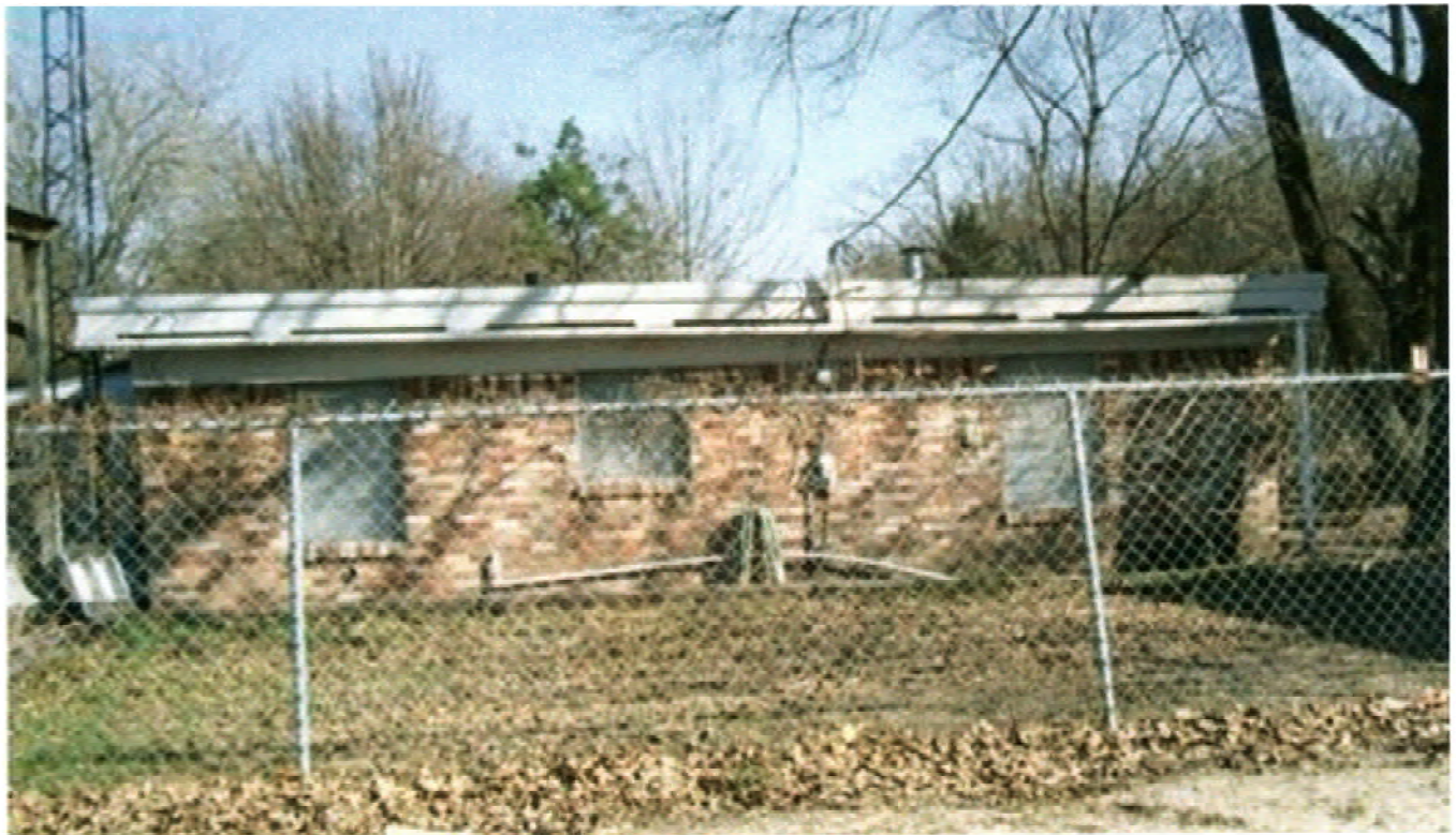
CLASS 1M LOW QUALITY MASONRY
