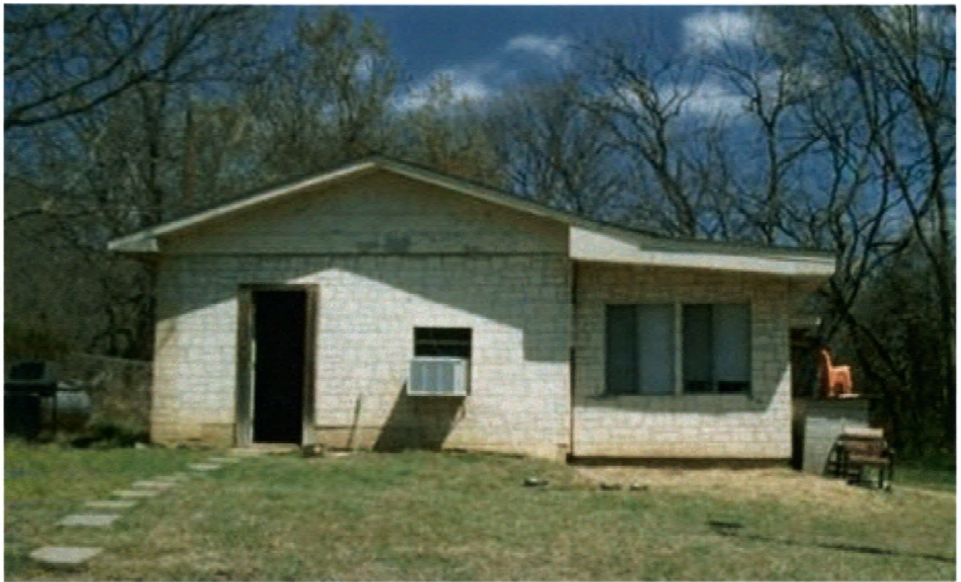
CLASS 1M LOW QUALITY MASONRY
